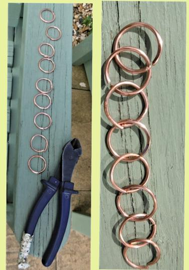
When completed, my 5 lengths of scrap copper wire made 106cm of chain, which was plenty long enough. All that remains to be done now, is to devise an end cap for the gutter that will allow the chain to hang a little further away from the greenhouse frame. (suggestions very welcome)
